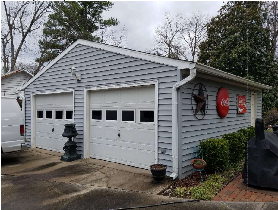
Existing Garage: View from House Back Door
