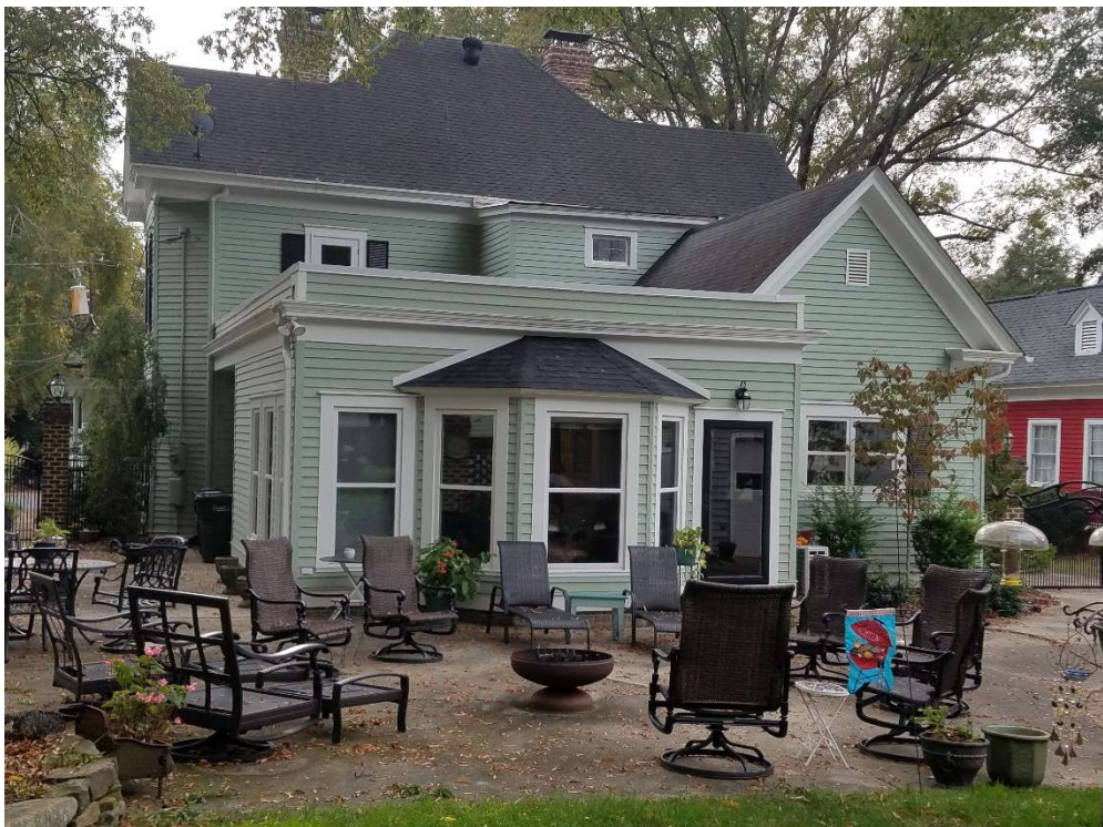
View of 2016 Addition & Back of House from Back Yard
